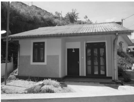
Figure 4: View of a sample house (Figure: 5) while the other three walls were proposed to be painted in brilliant white (Figure: 7, 8, 9). This decision ensured that the two rooms to be tested are identical in every aspect other than the introduced red or blue colour.
